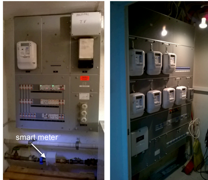
Figure 1: Two typical installations in the Swiss case study: single family (left) and multi-family (right).
